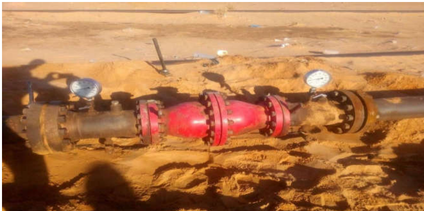
Figure III.12 :L'installation d'ENMAX du surface.
