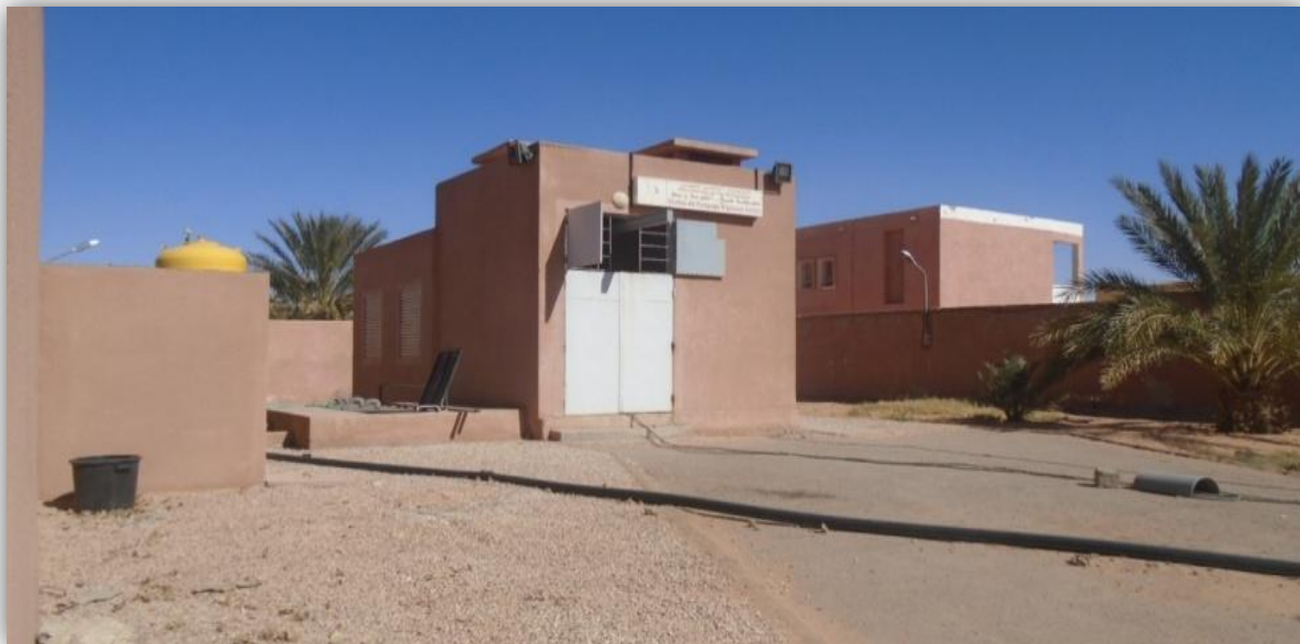
Photo (02): Station de pompage.
