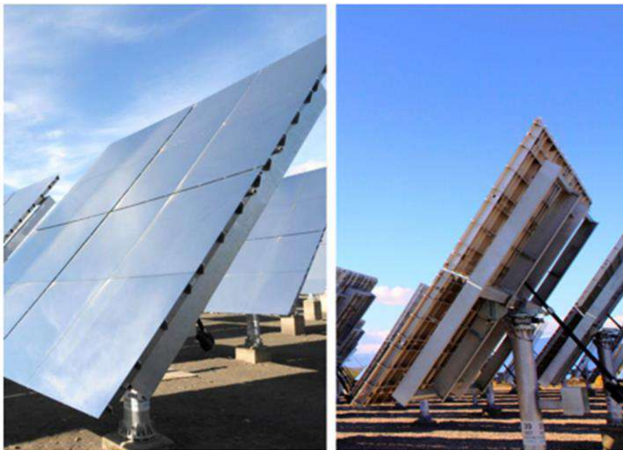
Figure I-16: AORA Solar heliostat with grid support structure and square torque tube.
