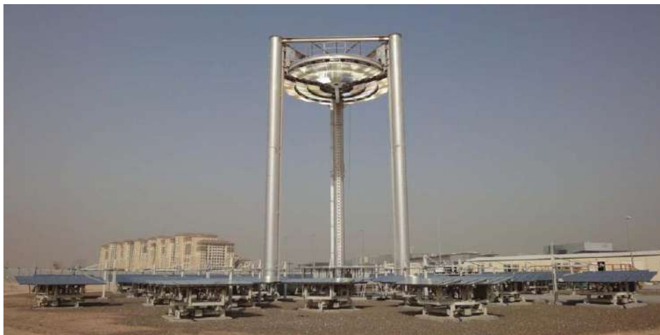
Figure I-10: Beam Down Solar Thermal Concentrator
