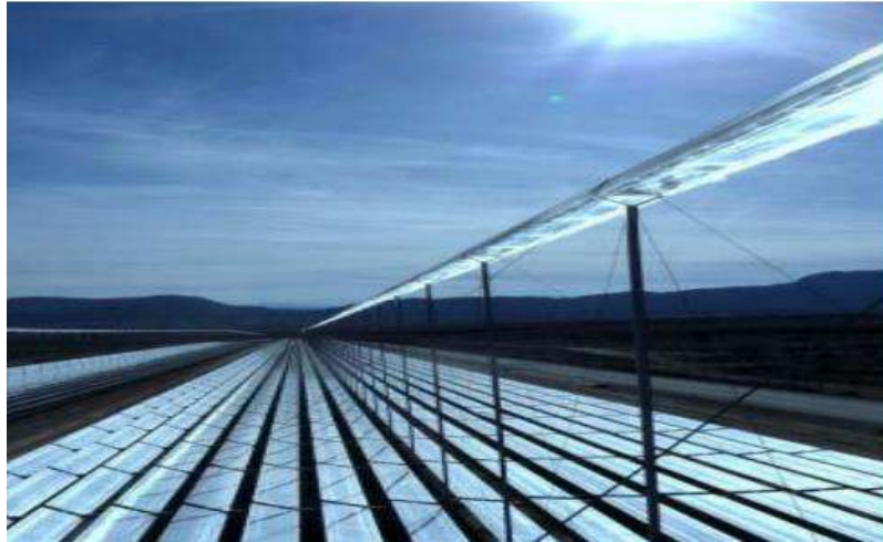
Figure I-8 : Linear Fresnel Solar Concentrator
