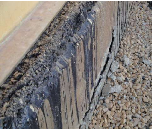
Figure II. 17 : Infiltration d'eau [11]
