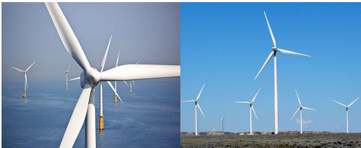
Figure I.11: High speed propeller type wind machines
