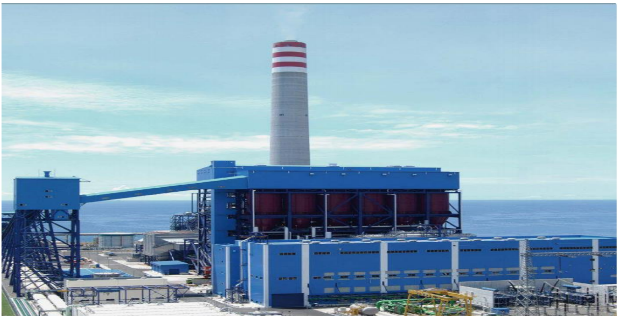
Figure I.13: Steam power plant
