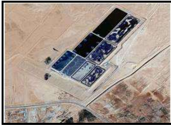
FIGURE (IV-3): la station d'épuration Ouargla.
