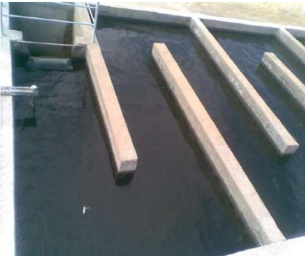
Figure III.20 Bassin de chloration
