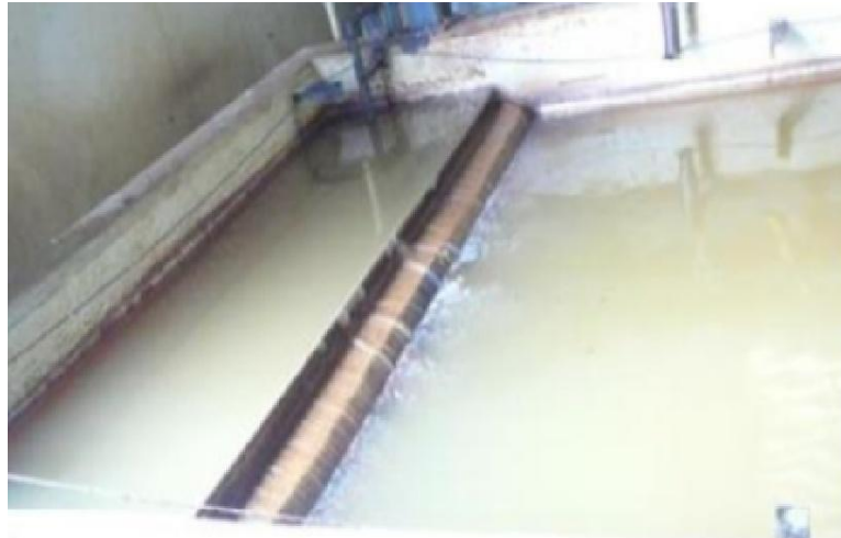
Figure I.4: CPI (Corrugated Plate Interceptor) [8]
