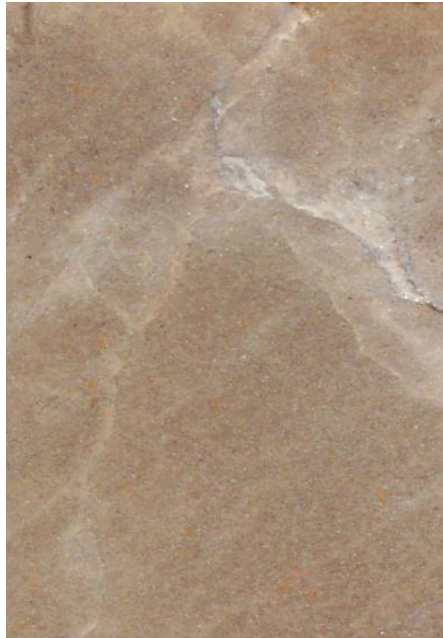
Figure IV.2: Typical Upper Zone Shear Fractures.[24]
