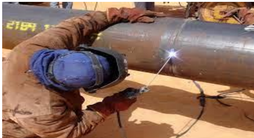
Figure III.1 soudure pipeline MIG [39]
