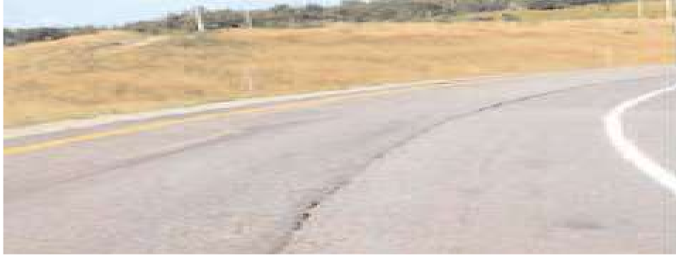
(figure II.14) Joint ouvert
