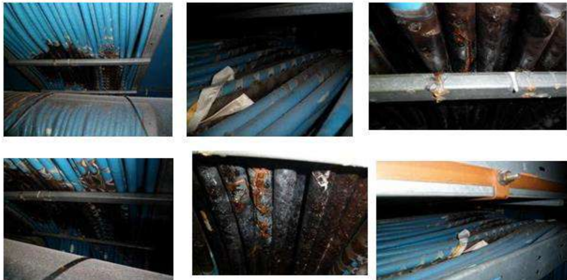
Figure I.12: Locally damaged cables. [20]
