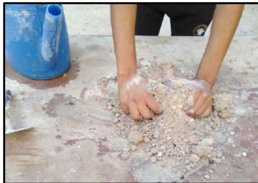
Figure III.2 Malaxage de Timchemt.
