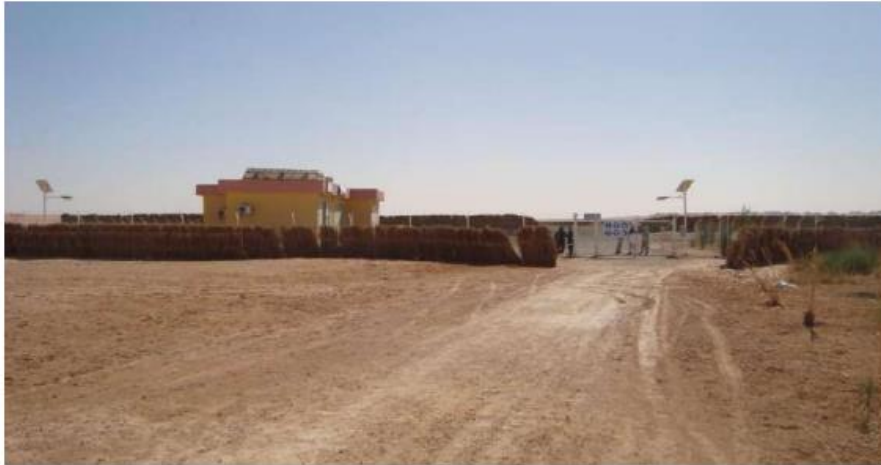
Figure III.11 Station d'épuration de N'goussa
