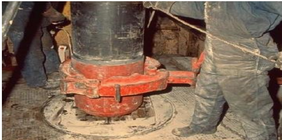
Figure II.28 : Sabot de tubage.
