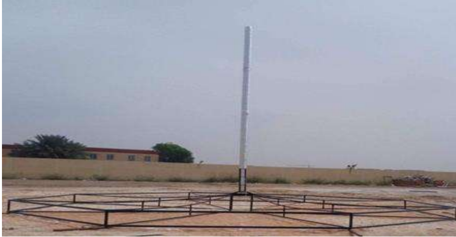
Figure III-3: A picture of the chimney.
