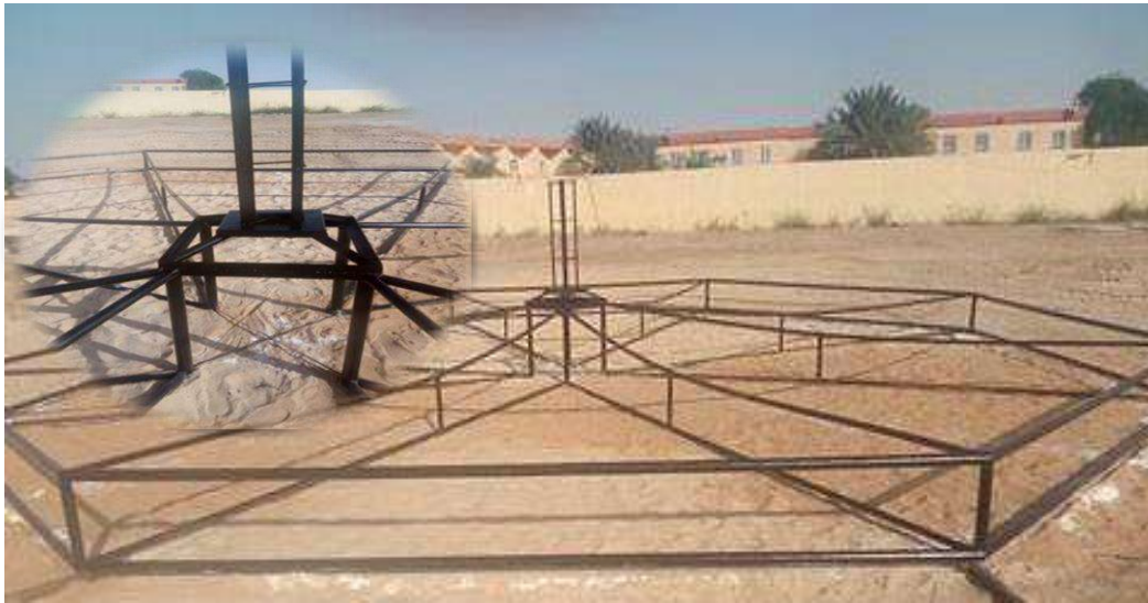
Figure III-4: Metal structure of the chimney.
