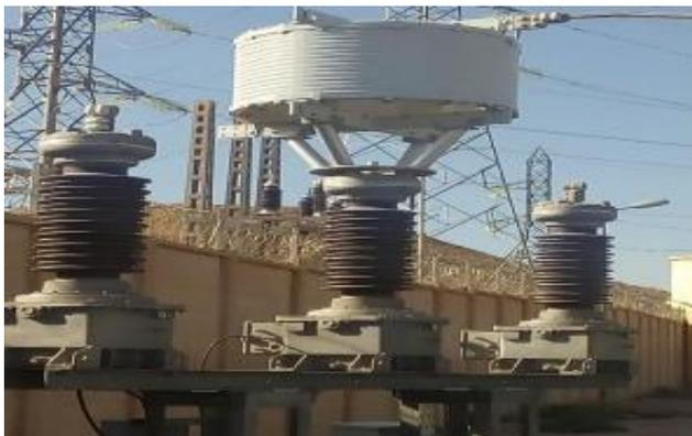
Figure II-5- le circuit bouchon (CB)[6]
