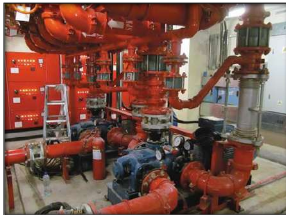
FIGURE 8: Multistage Multiport Pump.
