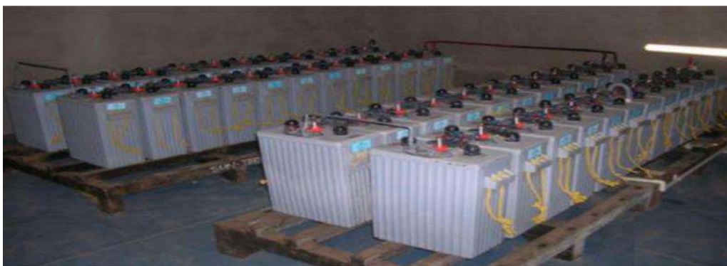
Figure 1.7. Battery bank
