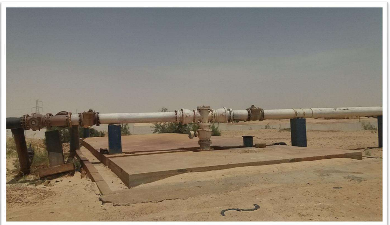
Figure I.4 : Forage ELMOSTAKBEL N°1
