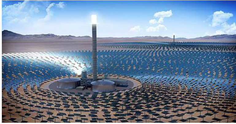
Figure I.7. Solar power tower with heliostats [10].
