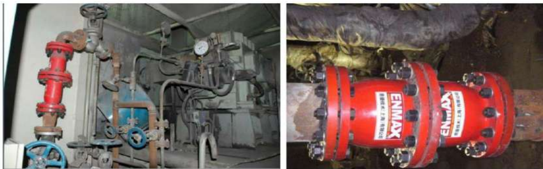
Figure I.48: Installation of ENMAX (Enmax Technology (Shanghai) Co, 2012).
