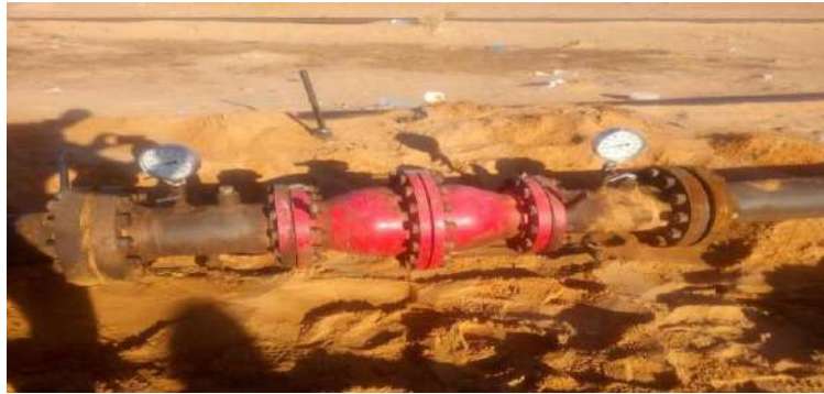
Figure I.57: Installation of ENMAX
