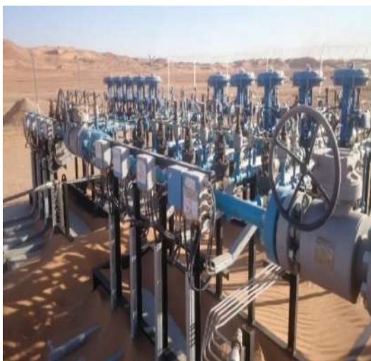
Control Valves of Wells
