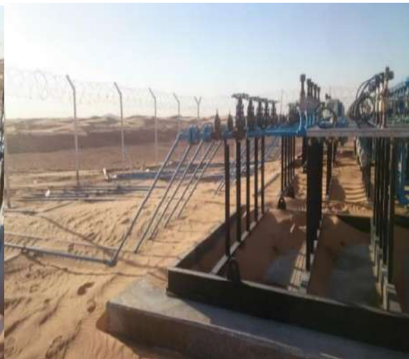
Control Valves of Wells
