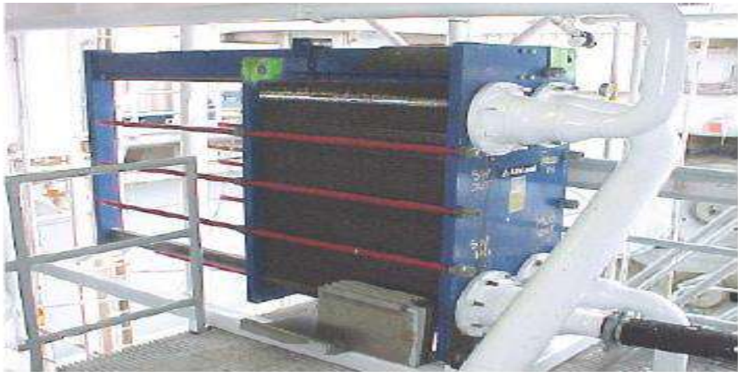
Figure III. 16 : mud cooler[5]
