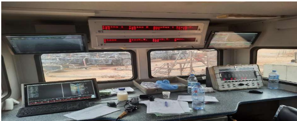
Figure II.14 CABINE DE CONTROLE. [24]
