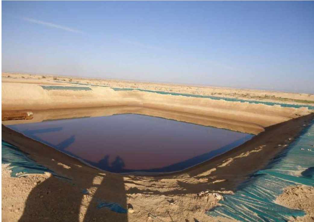
Figure 2: Dispositif passif (bourbier)
