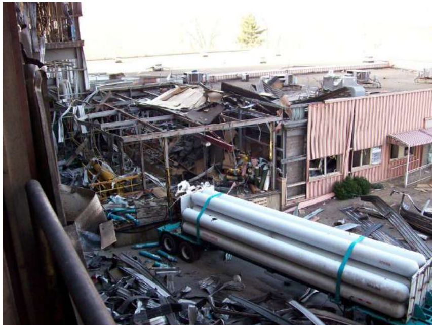
FIGURE 24 :FATAL HYDROGEN EXPLOSION AT A POWER PLANT IN MUSKINGUM, OHIO ,USA[10]
