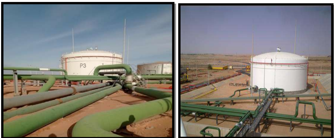
Figure III.7: The C4 Storage center
