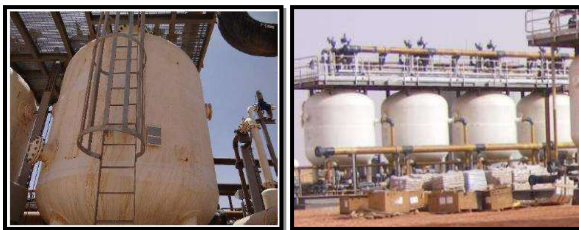
Figure III.16: Dual Media Filters WTC/ The NMWIC
