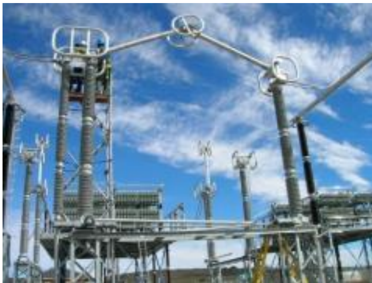
Fig I. 12 Disconnectors
