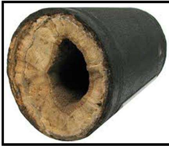
Figure (II.5): Calcium sulfate deposit. [7]
