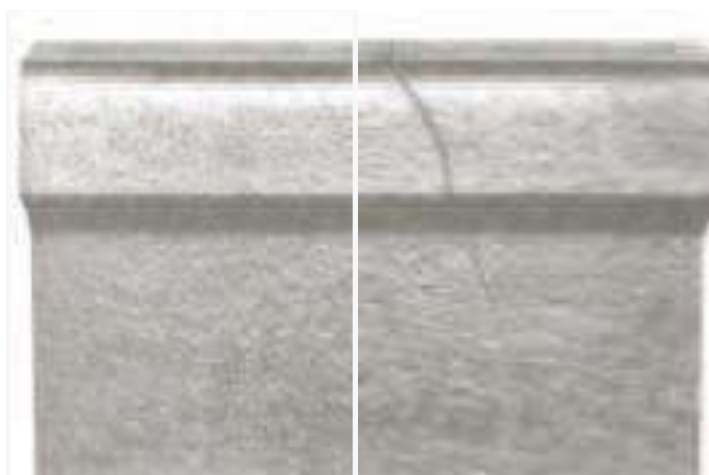
Figure I.5 : fissure des rail [8].
