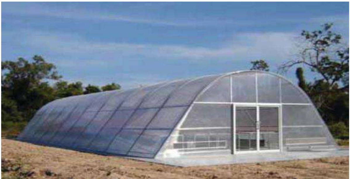
Figure II.8 Large scale solar dryer for polycarbonate greenhouse. [35]
