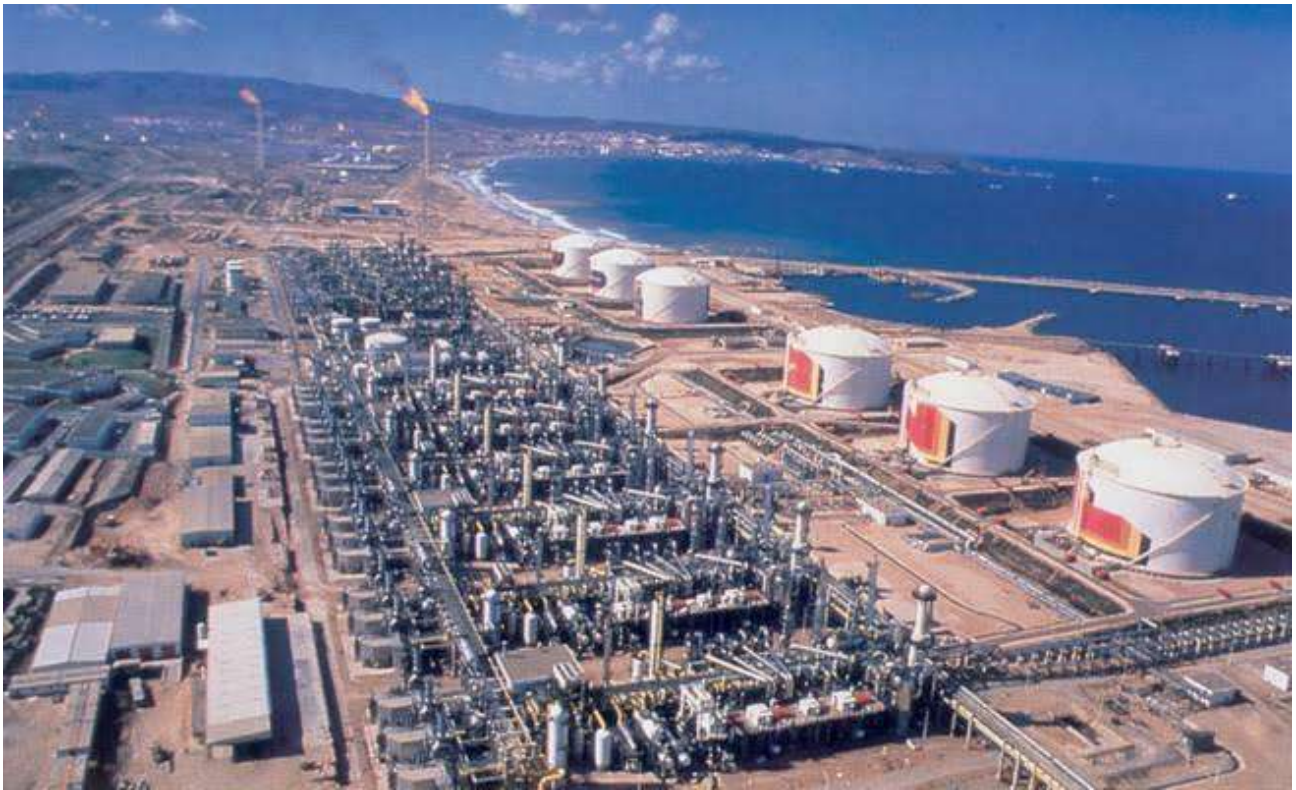
Figure 1 : station raffinerie des Arzew[3]
