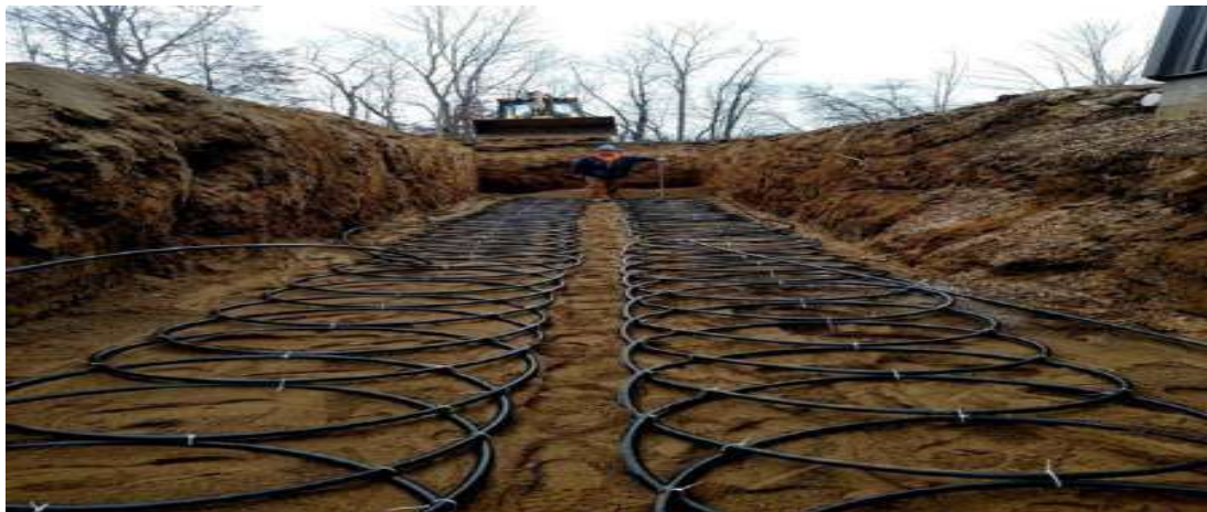
Figure I-1: Geothermal heat exchangers
