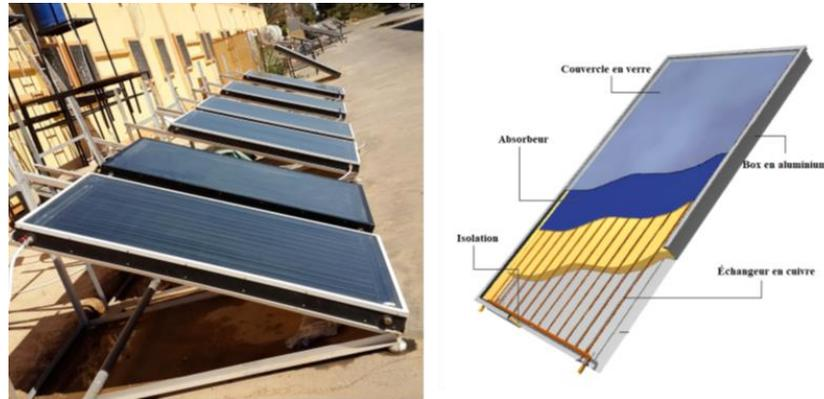
**Figure III 3. 9:chauffe-eau solaire CESTH 150 L commercial**
