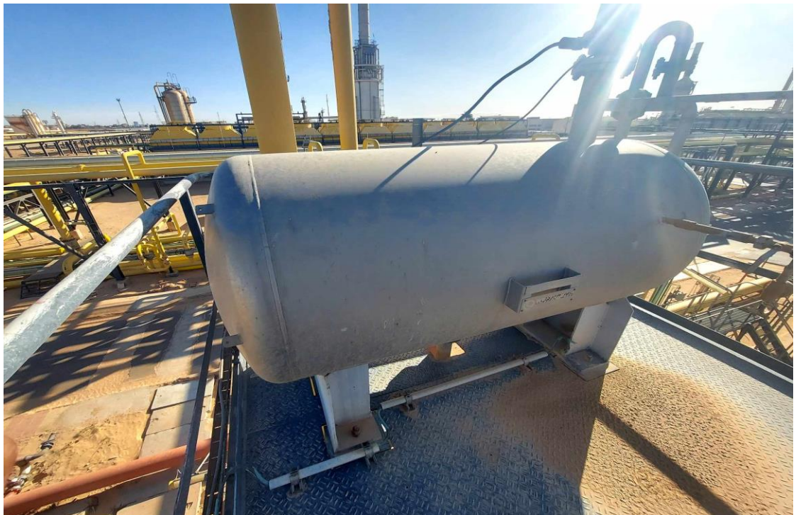
Figure 1-16 :ballon de graissage.
