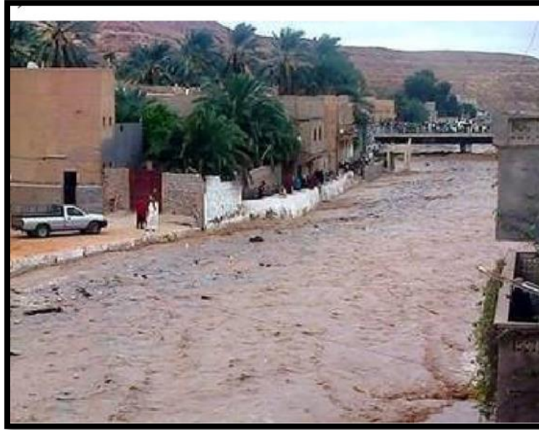
Figure 14. L’oued Metlili en crue (Crue 01 /10/2008 Debit max = 850 m 3 /s (Photo. Ouled)
