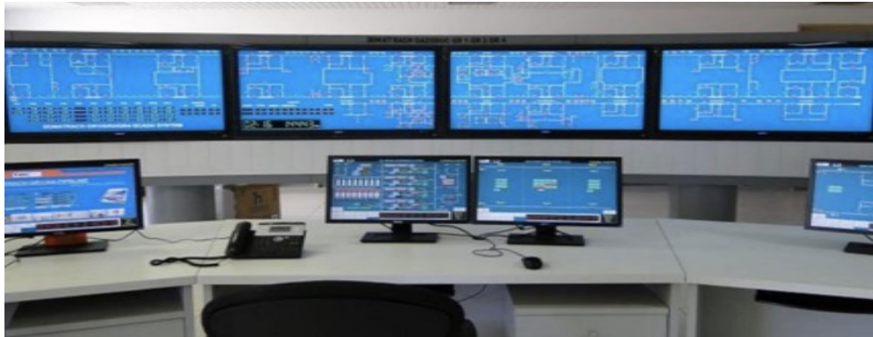
Figure II.5: Example of supervisory control and data acquisition [14]
