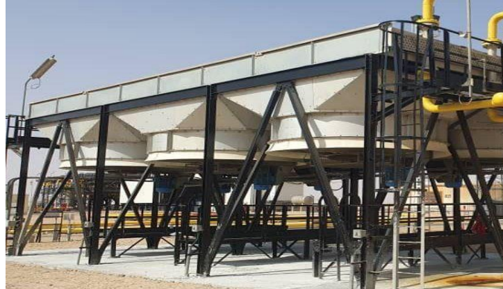
Figure 4 – Les Aerorefrigérant (EA-01/EA-02)
