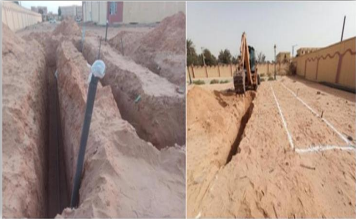
Figure III- 2: A general display of the system used for the cooling of photovoltaic panels.
