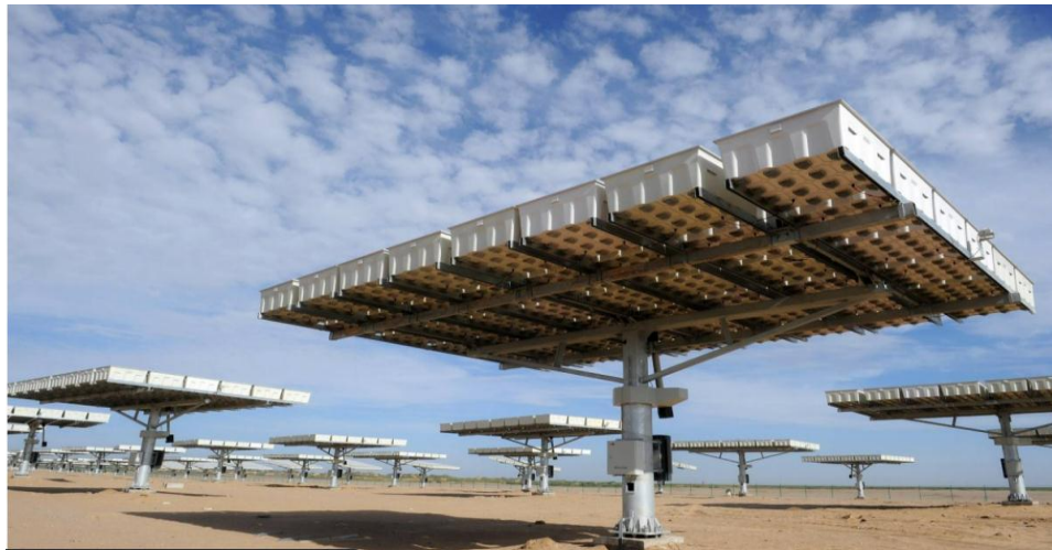
Figure I.29: CPV project in Golmud, China
