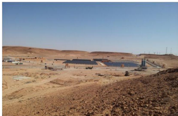
Figure I.30: photovoltaic power plant -Ghardaia- Oued Nechou [23].
