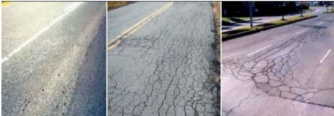
Figure 4: Examples of Crazing at Different Severity Levels.
