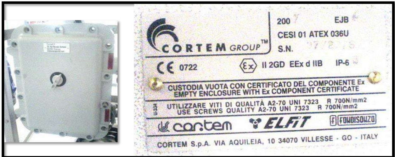
Figure III06 : Boite jonction ATEX.
