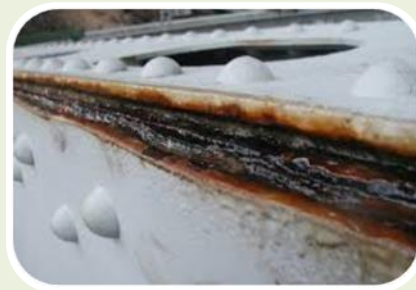
crevice corrosion
