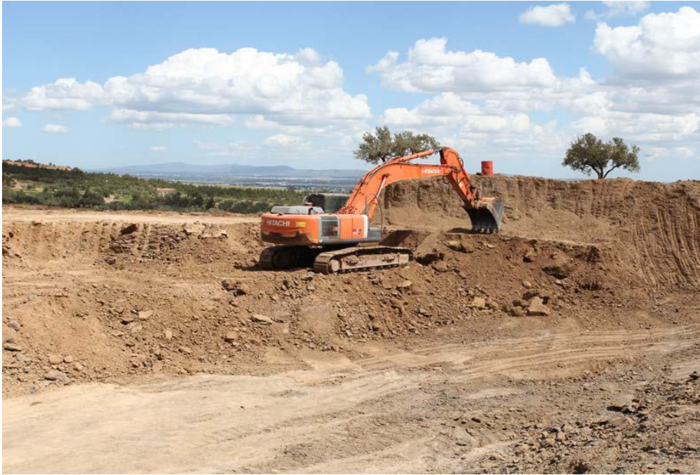
Figure II.2 : Extraction de l'argile [27]
