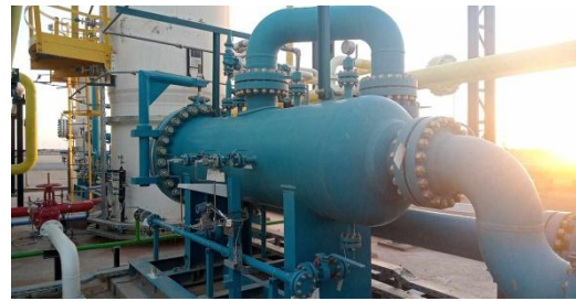
Figure IV.7: Guard Bed Filter
