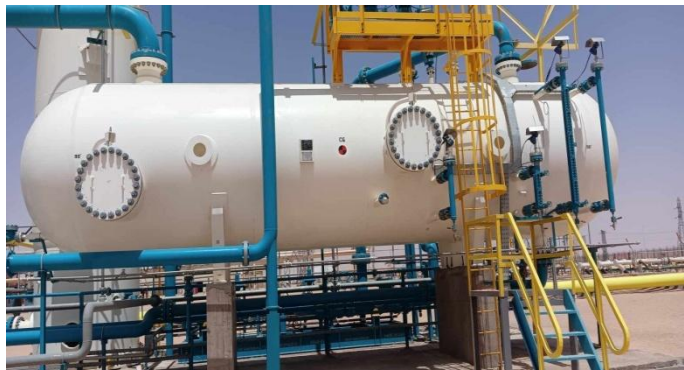
Figure IV.2 : Three Phase Separator
