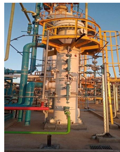
Figure IV.3: Filter coalescer
