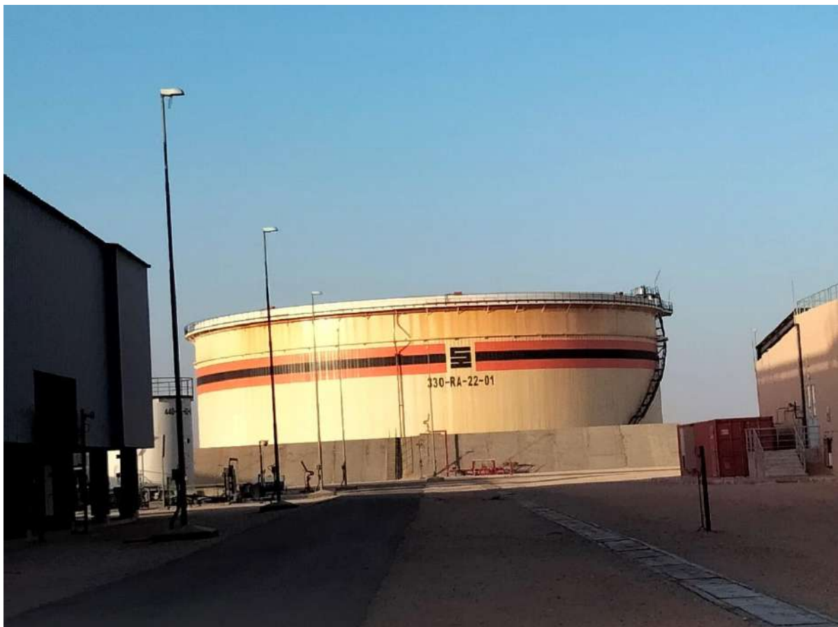
Figure I.12: Bac de stockage
