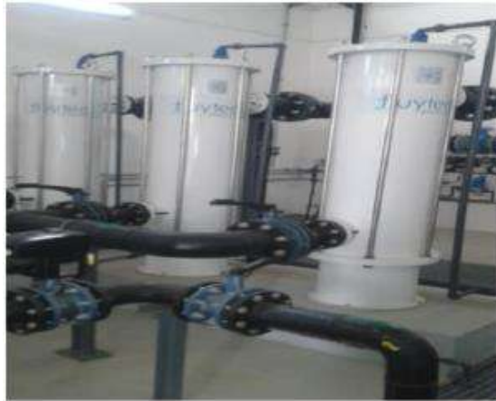
Figure III.8: les filtre a cartouche
