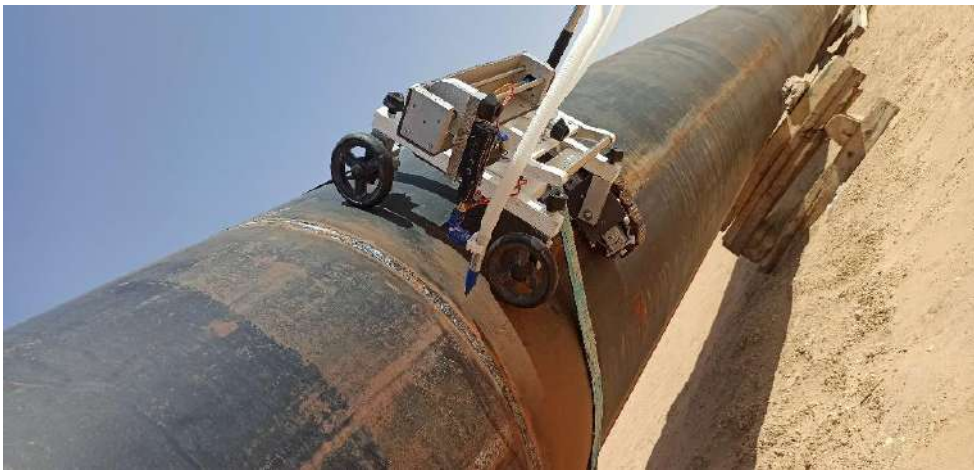
Figure 3.6: Robot welding method for gas and oil pipelines.
