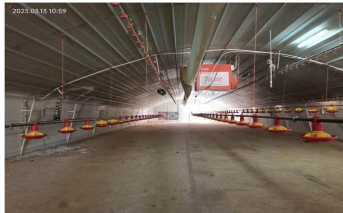
Figure III. 4: Real photo industrial poultry house Al-Hajjah Al-Tijani Farm Company for Poultry and Feed [50m]
