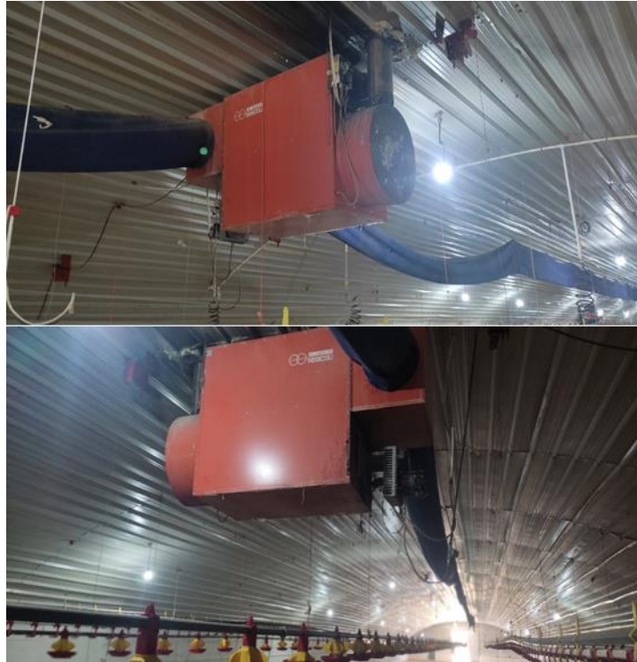
Figure III. 2: The combiTERM - indirect exchange hot air generator
