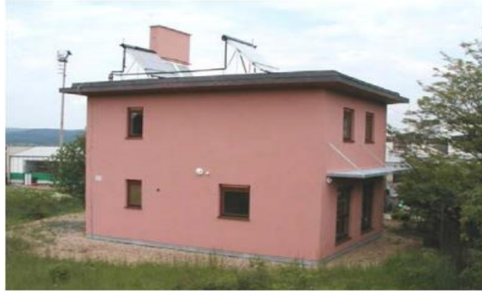
Figure II. 4: Experimental house with hybrid ventilation. (9)
