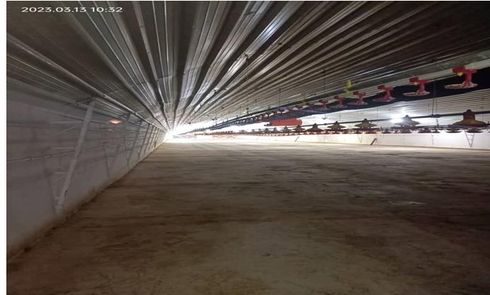
Figure III. 3: Real photo industrial poultry house Al-Hajjah Al-Tijani Farm Company for Poultry and Feed [120m]
