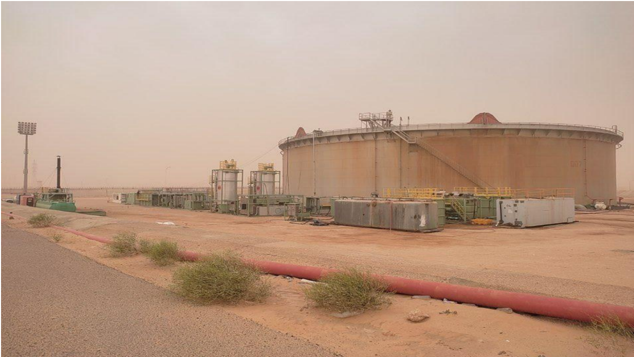
Figure III.1: Traitement ON-LINE (Bac de stockage OD7 Houde El Hamra SH)
